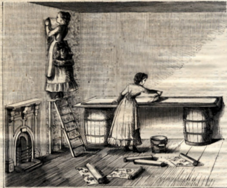
Fig. 3.—PASTING AND PUTTING ON WALL-PAPER.
